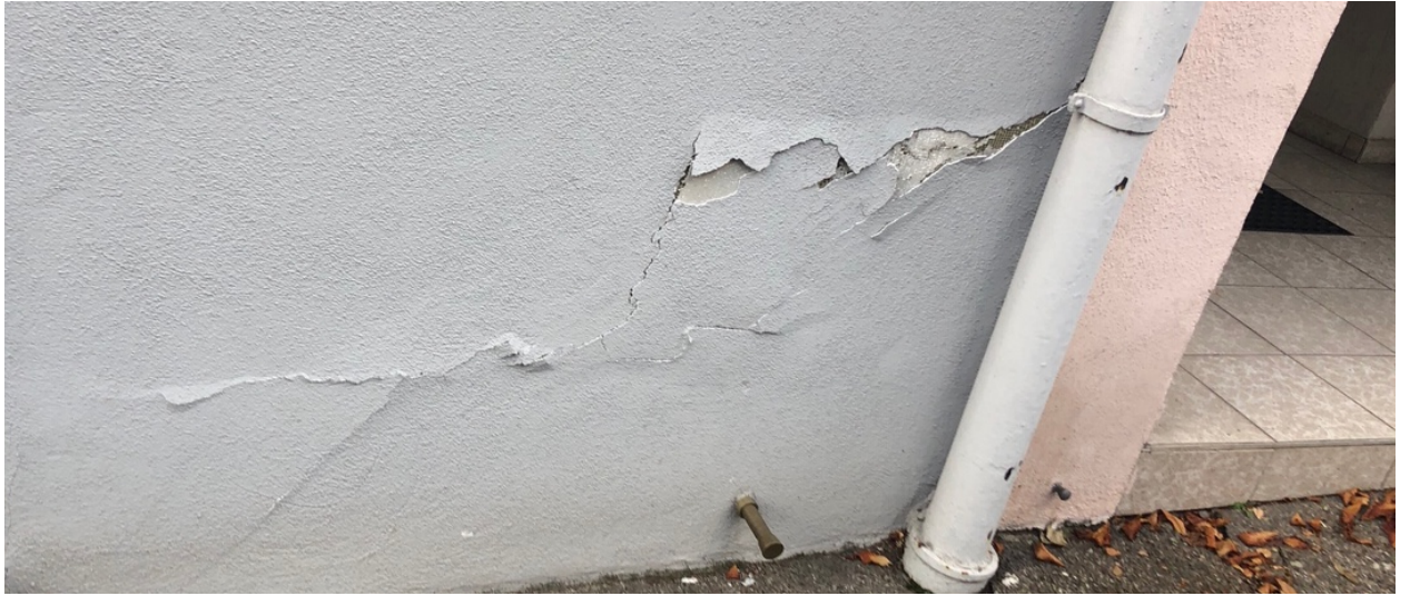
Figure 4.14: Cracks in the building started to appear at the same time (May 2019) as the observed release rupture in the time series (Fig. 4.13).
