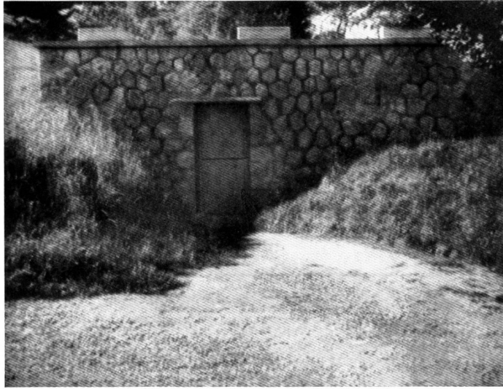
Station nouvelle cave no. 128
