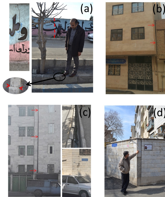
Figure 5.2.: Examples of damage caused by groundwater-induced compaction to the southwest of Tehran. Pictures (a)–(d) are associated with the locations in Figure 5.1 indicated by the blue, green, black, and red stars, respectively. We observed cracks in walls and the ground, shifts in curbstones, and tilted buildings at different locations. The pictures were taken in 2015 and 2017.
